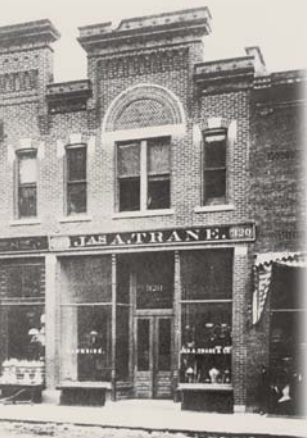
Trane Storefront La Crosse, Wisconsin 1891
